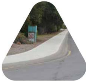
Kerbs & Footpaths $.91 million
