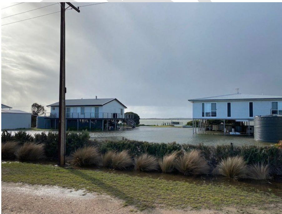
Flood waters surround properties along Mundoo Channel, April 2023 (Photo B Wright)
