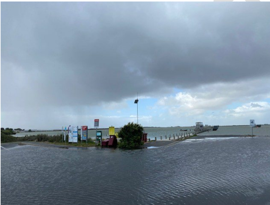
Flood waters over the Mundoo Channel car park and boat ramp, April 2023 (Photo: B Wright)
