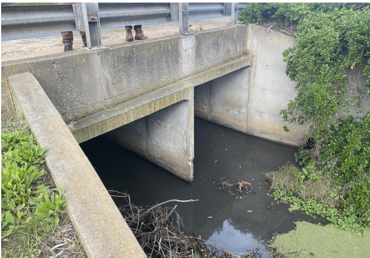
Figure 2-3: Goolwa Road culverts (upstream side)
