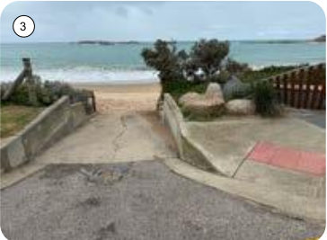
Boat ramp no longer required, opportunity to provide ramped pedestrian access to the beach
