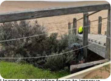
Upgrade the existing fence to improve public safety
