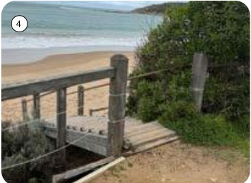
Opportunity to demolish and reconstruct Stair No. 4 to align with Stair No. 1, creating a clear pathway from Basham Parade to the beach
