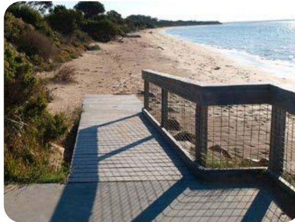
DDA access ramp to beach Point Nepean, Melbourne Australia
