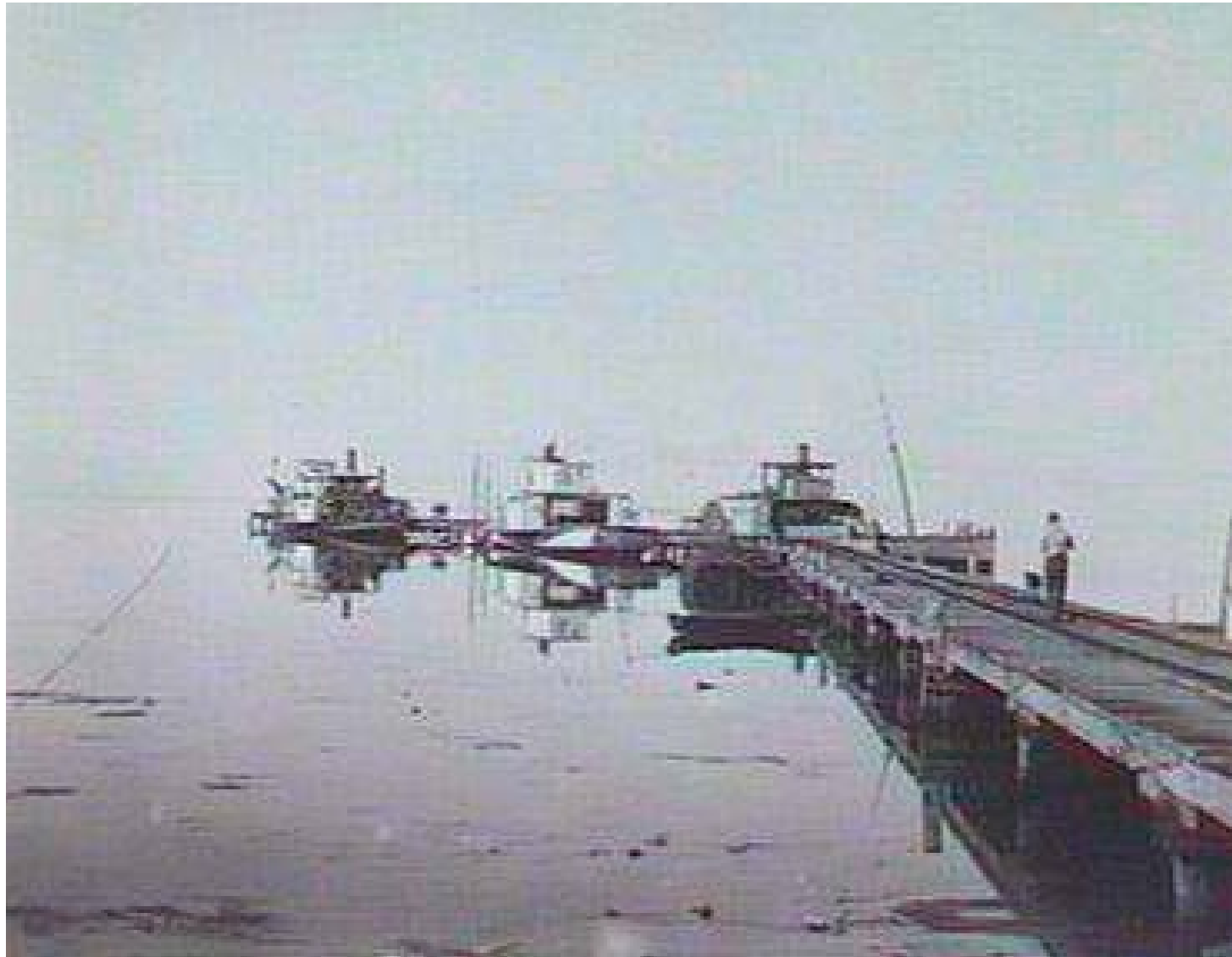
Photo of Milang jetty circa 1900. Construction of the 220 feet jetty began in 1856 and was extended to 711 feet in 1859 to support increase shipping and changing water heights. The township was a thriving port between 1860 to 1880 (Source McDougall & Vines Conservation and Heritage Consultants 2015)
