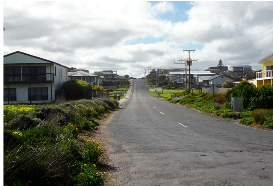
Photo of Chapman Road and Middleton's change in elevation
