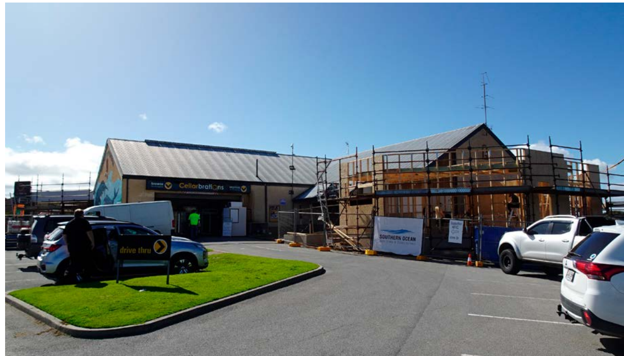
Middleton Tavern currently undergoing renovations
