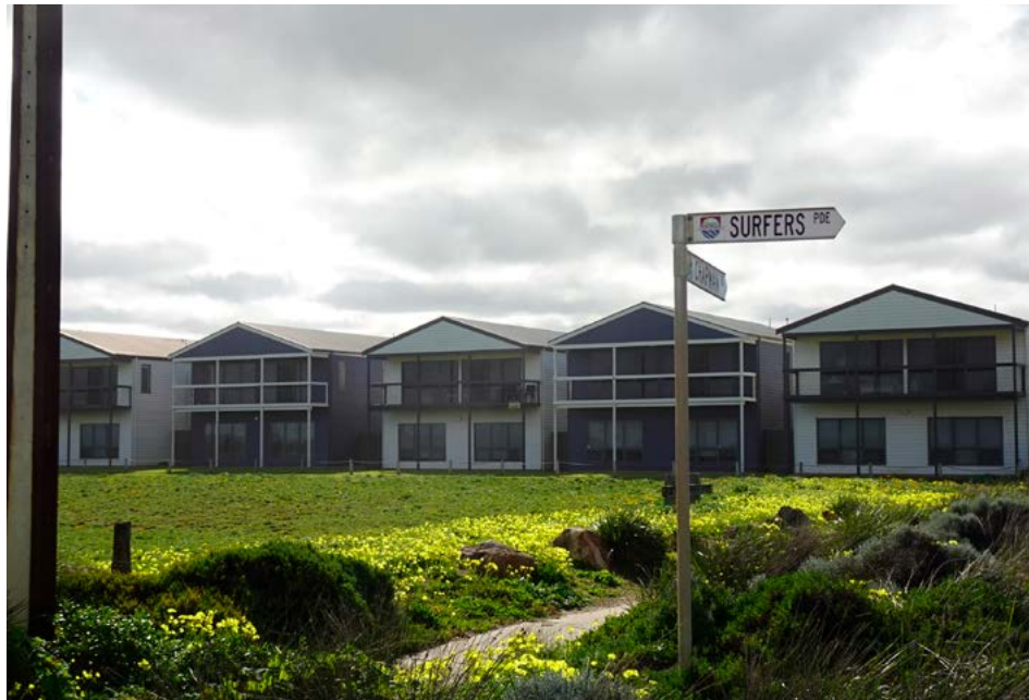
Dwellings facing onto Middleton Beach and overseeing Roscrow Reserve
