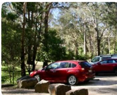
Roadside parking with rock boulders to identify parking bays and provide safety measure or alternative bollards
