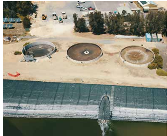
Wastewater treatment plant, Goolwa
